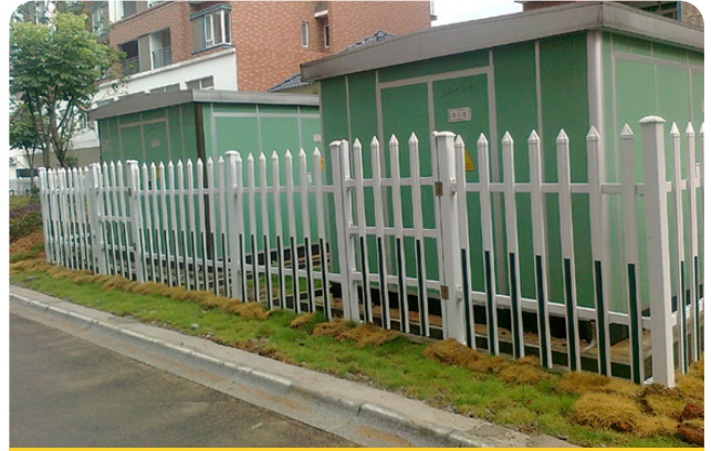
Power Station Fencing
